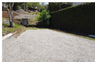
Rainpark G. Cariari, Belén, Flood control
